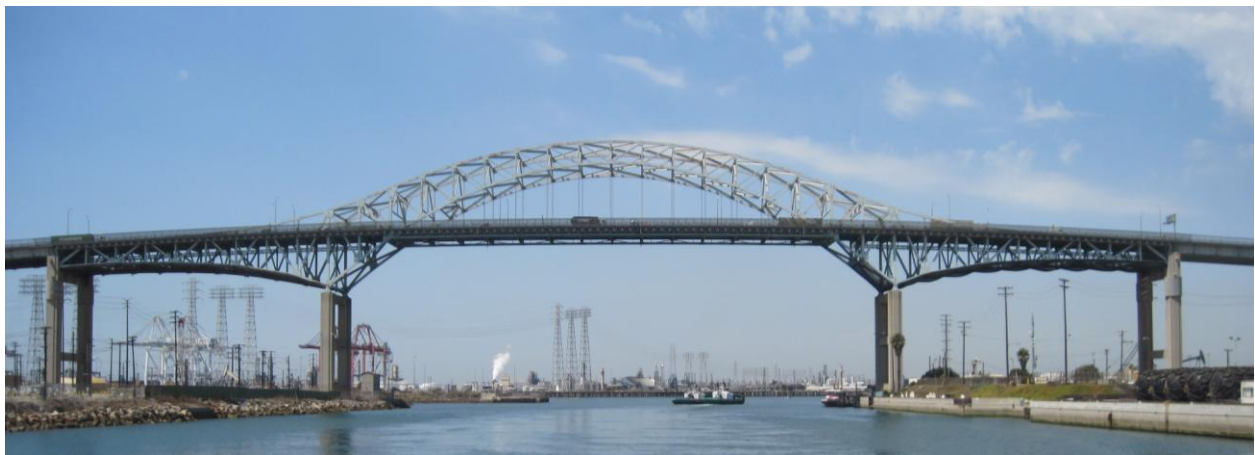
FIGURE 46. GERALD DESMOND BRIDGE, PORT OF LONG BEACH
