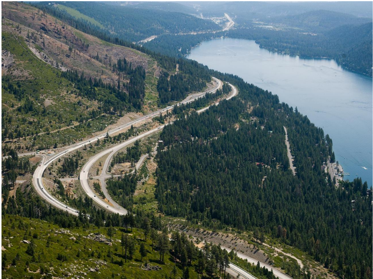
FIGURE 4. INTERSTATE 80 AT DONNER PASS – TIER 1 FREIGHT HIGHWAY DESIGNATION
