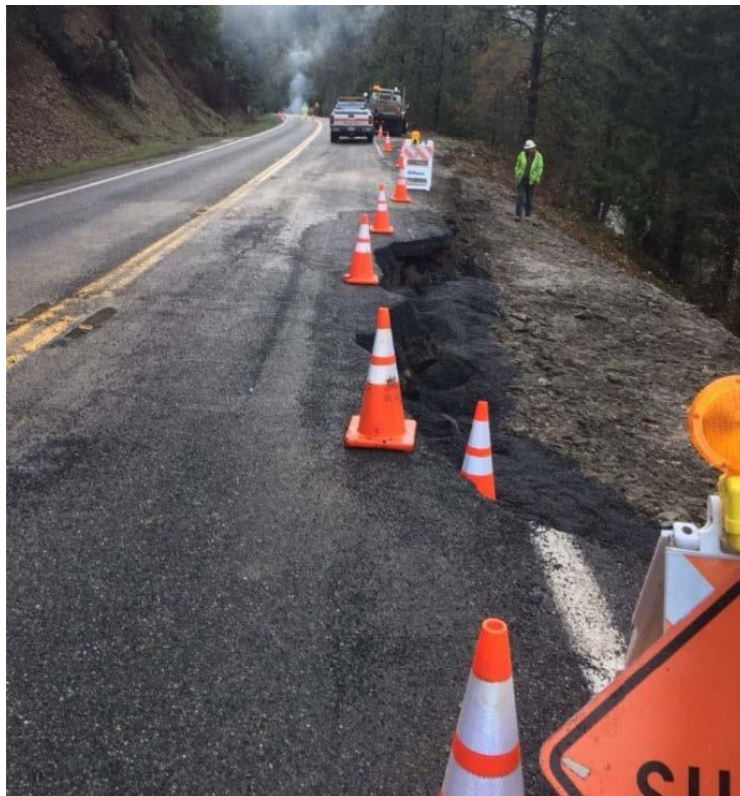
FIGURE 6: EROSION ON SR 96 NORTH OF SOMES BAR
