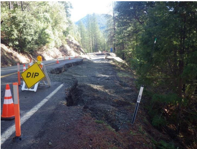
FIGURE 3: PLUMAS STATE ROUTE 70 STORM DAMAGE IN AN AREA KNOWN AS THE "GAUNTLET"
