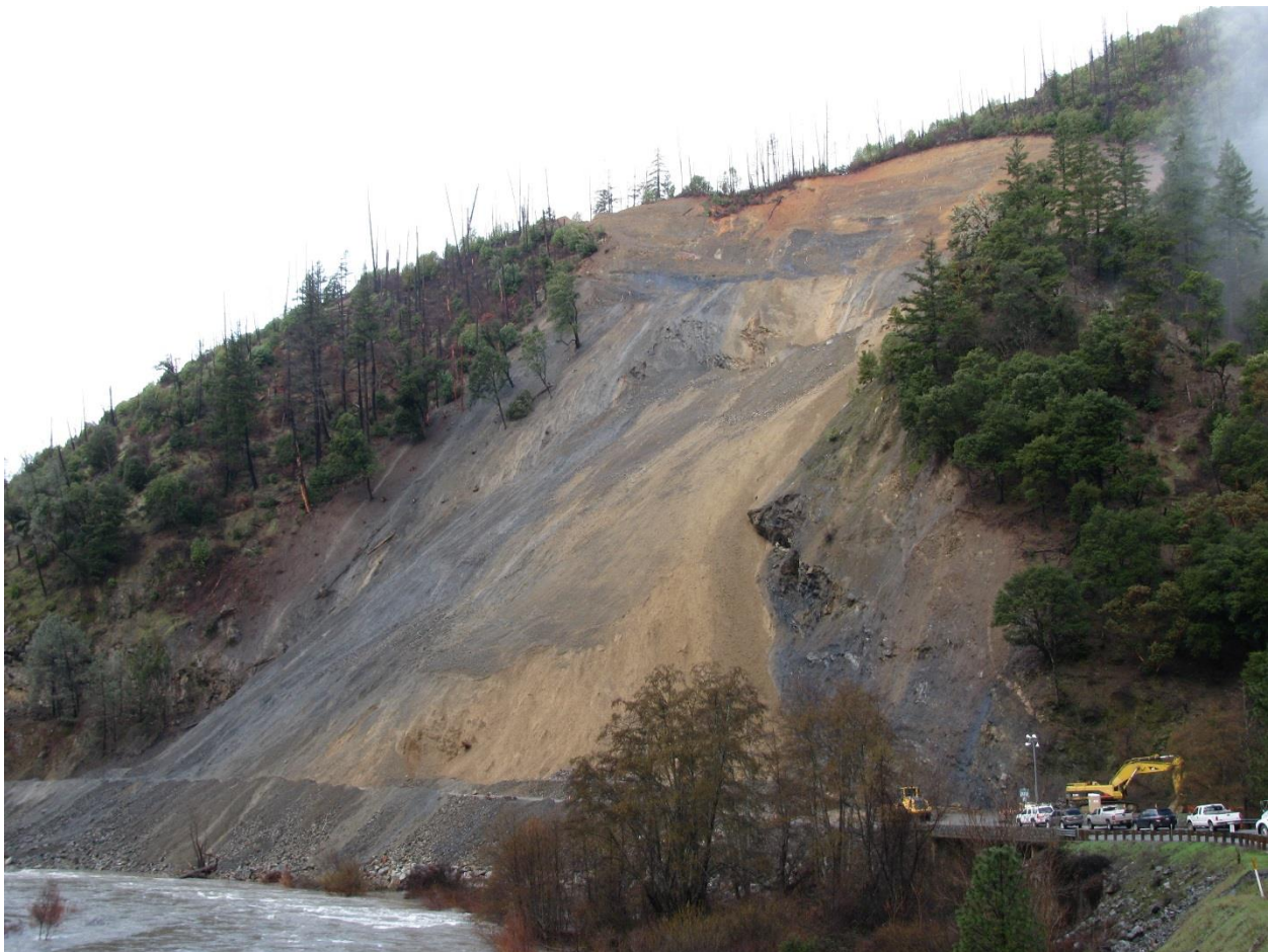
FIGURE 24: FACE OF THE BIG FRENCH CREEK SLIDE COMPROMISED AFTER HEAVY RAINS
