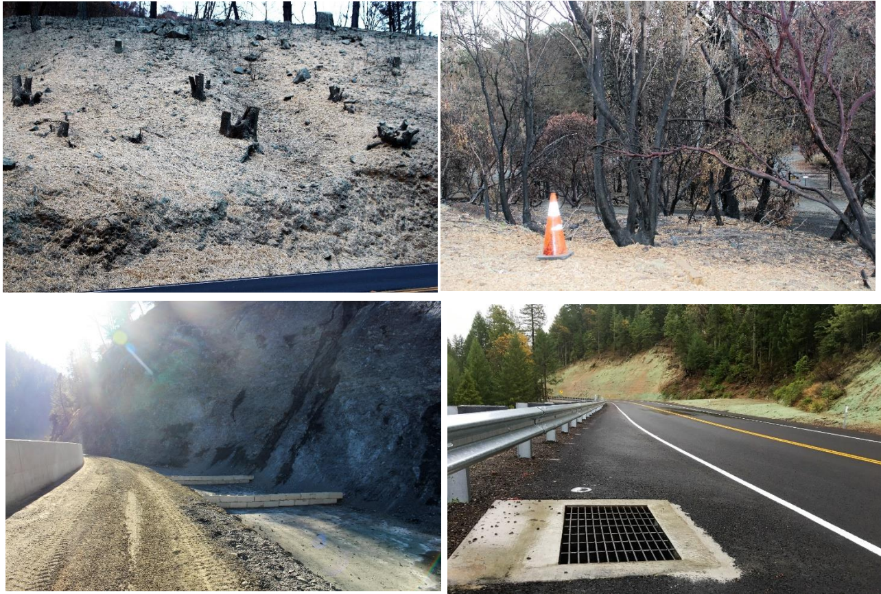
FIGURE 27: IMAGES OF HYDRO SEEDING AND NEW INFRASTRUCTURE AFTER THE HELENA FIRE
