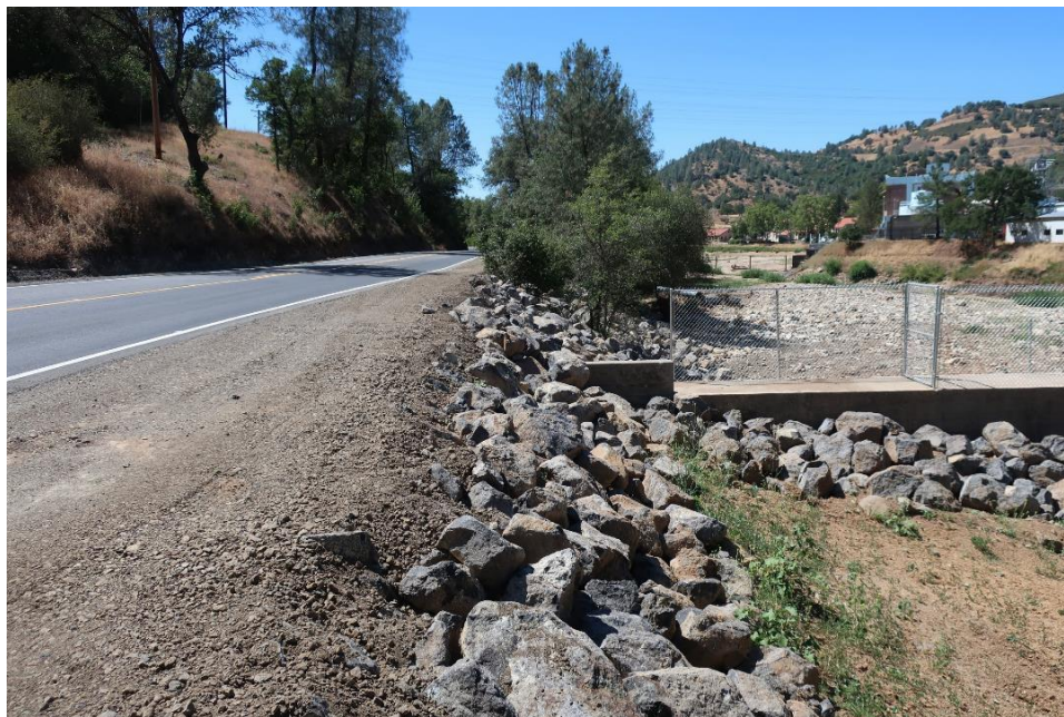
FIGURE 27: REPAIRED ROADWAY SR 49 IN TUOLUMNE COUNTY, MAY 2018
