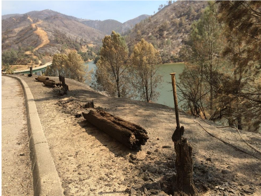
FIGURE 4: DAMAGE FROM THE DETWILER FIRE
