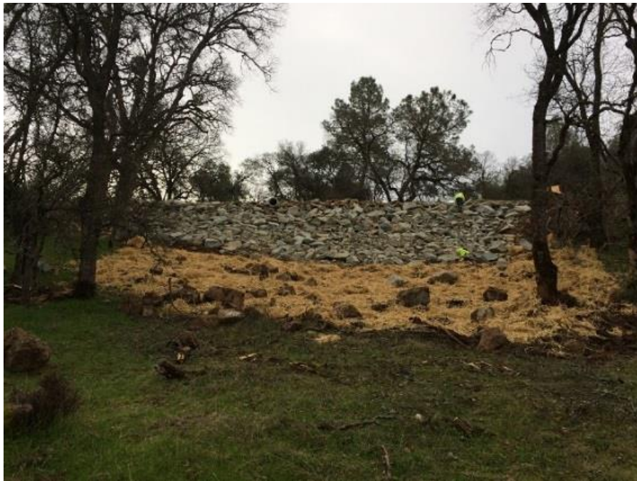
FIGURE 3: EXAMPLE OF LANDSLIDE REPAIR WORK ON SR 26
